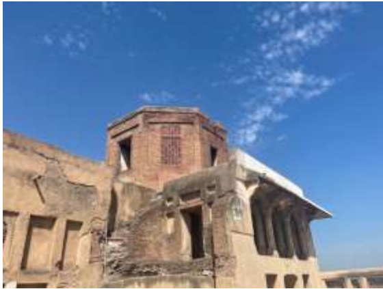
Figure 18 Southern elevation of the Kala Burj.
