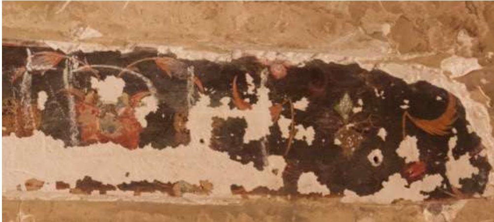
Figure 16 Western chamber. Painted panel. Flaky painted layer hidden behind thick plaster. Detailed floral study.
