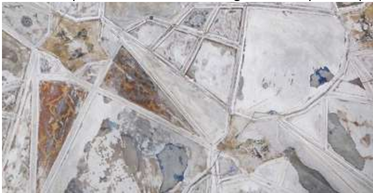
Figure 31. Kala Burj dome. Underpainting visible under final paint layer.
