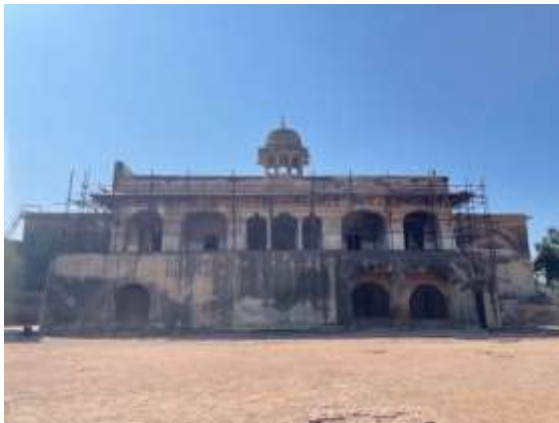
Figure 35 North-facing elevation of the DKKOA. Akbar period, with restoration work.
