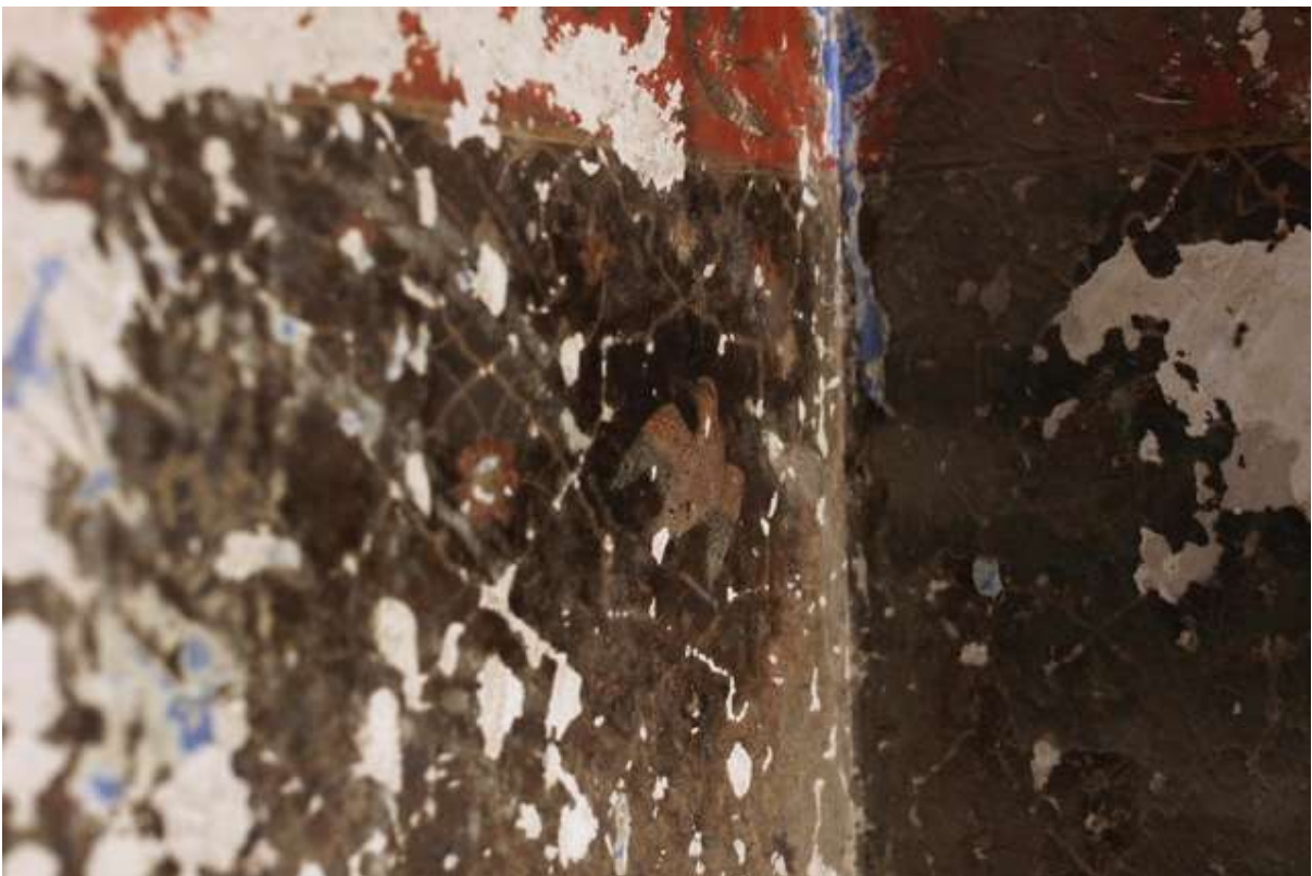
Figure 22 Detail of northern entrance first floor. Painted geometric pattern on dado, with birds. Blue layer visible.
